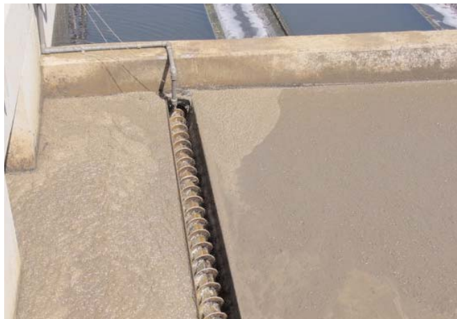
Scum Collector with travelling conveyor
