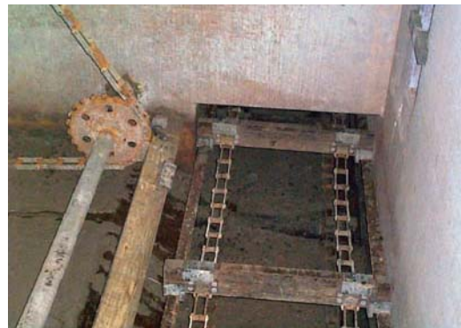
2 systems of grit chamber scraper apparatus applications
