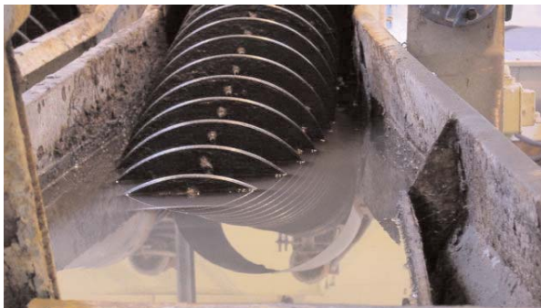
Screw Conveyors used for Grit Removal
