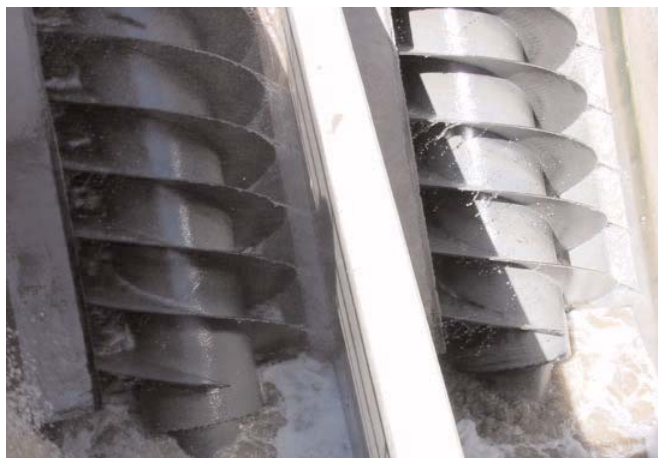
Screw lift pump with bottom bearing submerged in abrasive slurry
