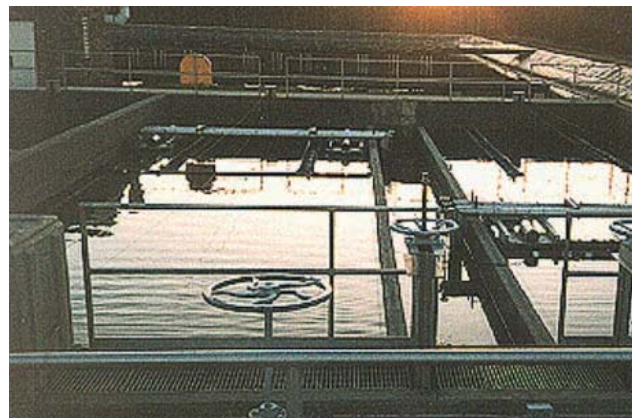
Primary Clarifier/Settling Tank
