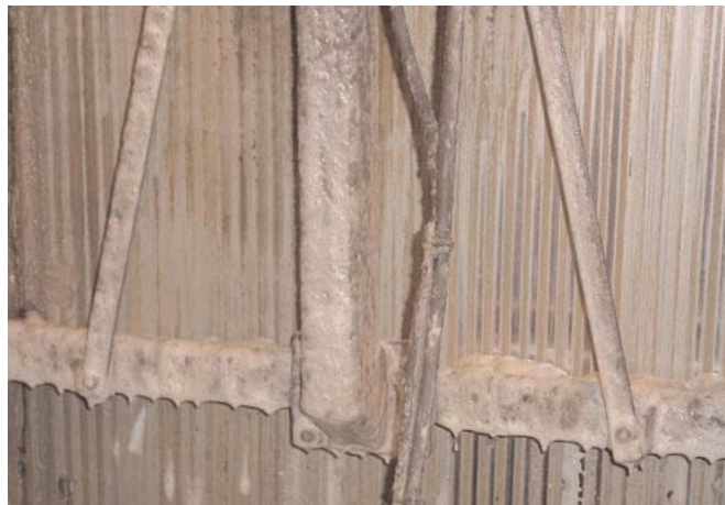
Bar Screen with Rake
